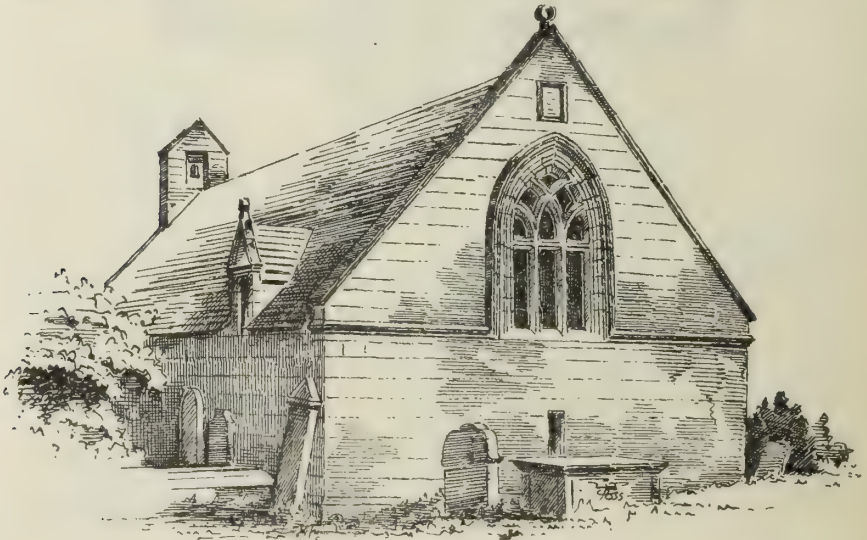
FIG. 1609.—Walston Church, showing Dormer.
